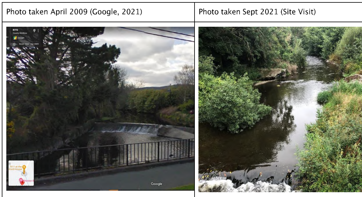
Figure 4-2: Ashford weir 2009 vs 2021
